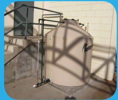
- new water reuse tank
