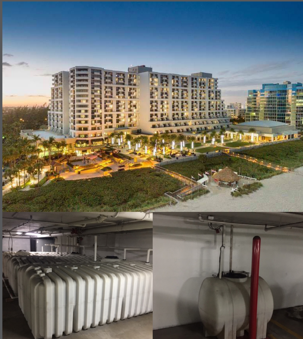
Cistern Tank Used for Capturing Rain Water, Harbor Beach Marriott Resort & Spa , Florida, USA
